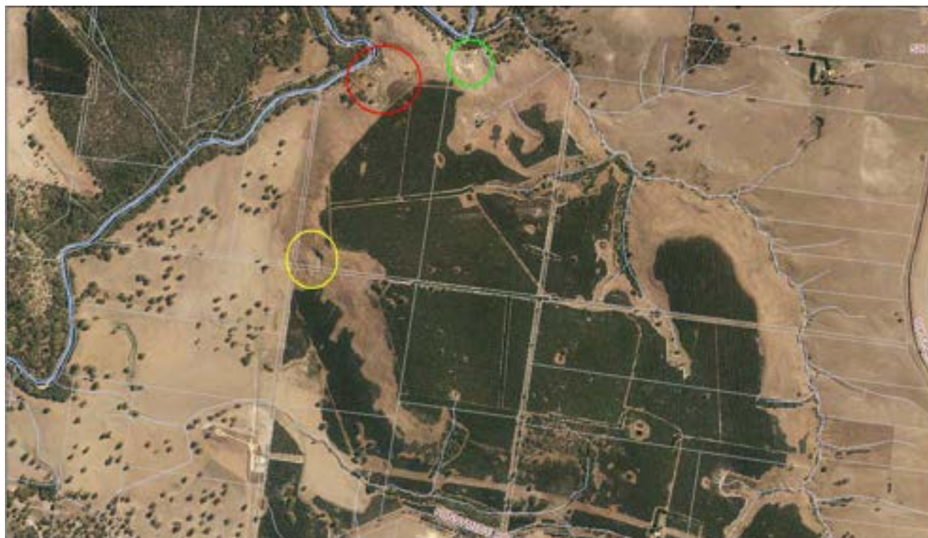
Photo 15: Locations of Landslips at Runnymede using 2010 imagery. Comparison of aerial photos shows landslips have not significantly changed since at least 1953.
